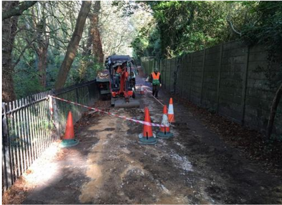
Figure 3: Conservation Team undertaking repairs to Millfield Lane
